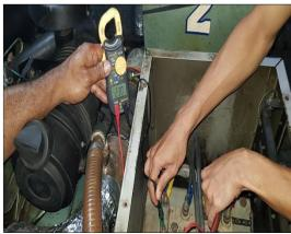
Fig. 5. Check the generator output voltage with neutral
