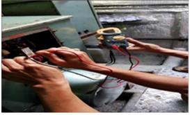
Fig. 6. Voltage check on AVR
